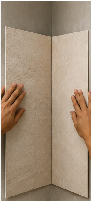
3 TWO PANELS – INTERIOR CORNER
