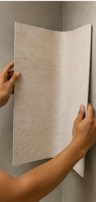
1 DRY FIT – INTERIOR CORNER
