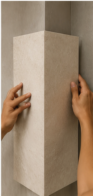
2 WRAP INTO INTERIOR CORNER
