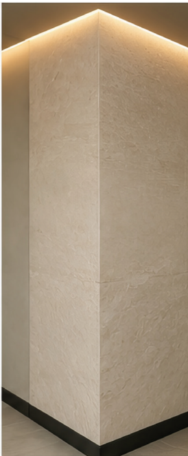
6 FINISHED CORNER INSTALLATION
